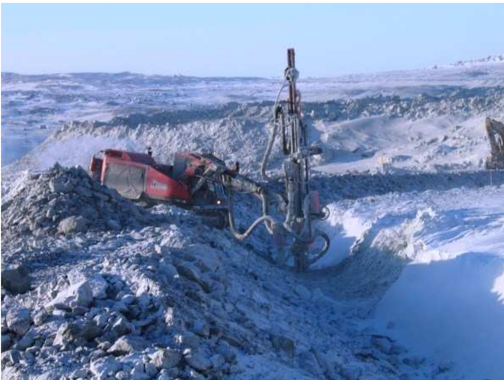
Photo 7: Drill working in key trench
