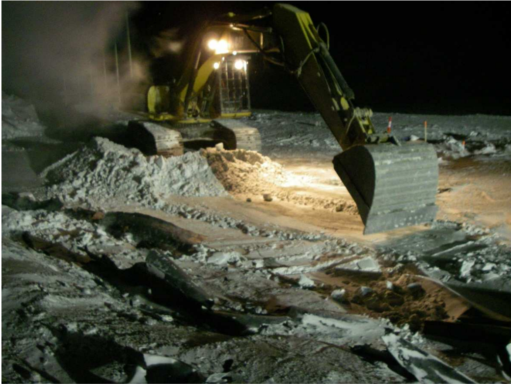
Photo 8: Removing snow from the south end of the dam, on the upstream side.
