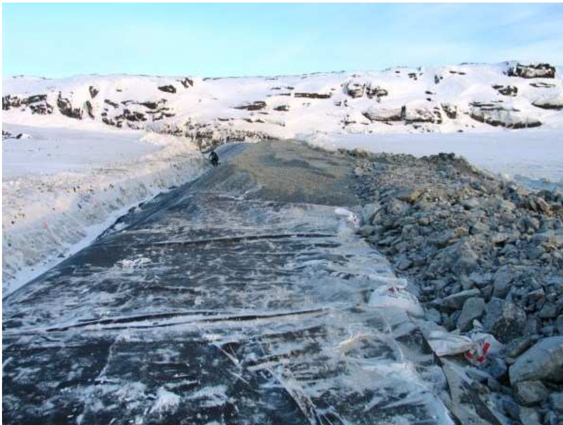
Photo 5: Start of modifications to the surface of the berm to permit equipment access. Sta. 580
