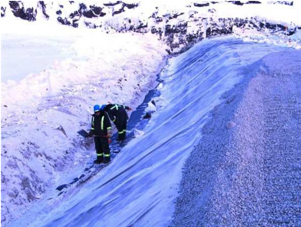
Photo 6: Labourers removing snow in key trench.
