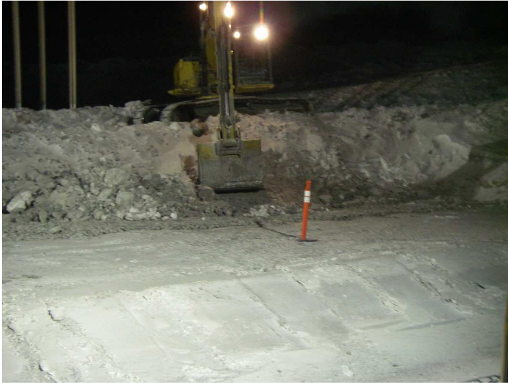
Photo 10: Excavator placing ROQ around Sta. 1+90, downstream of the core.
