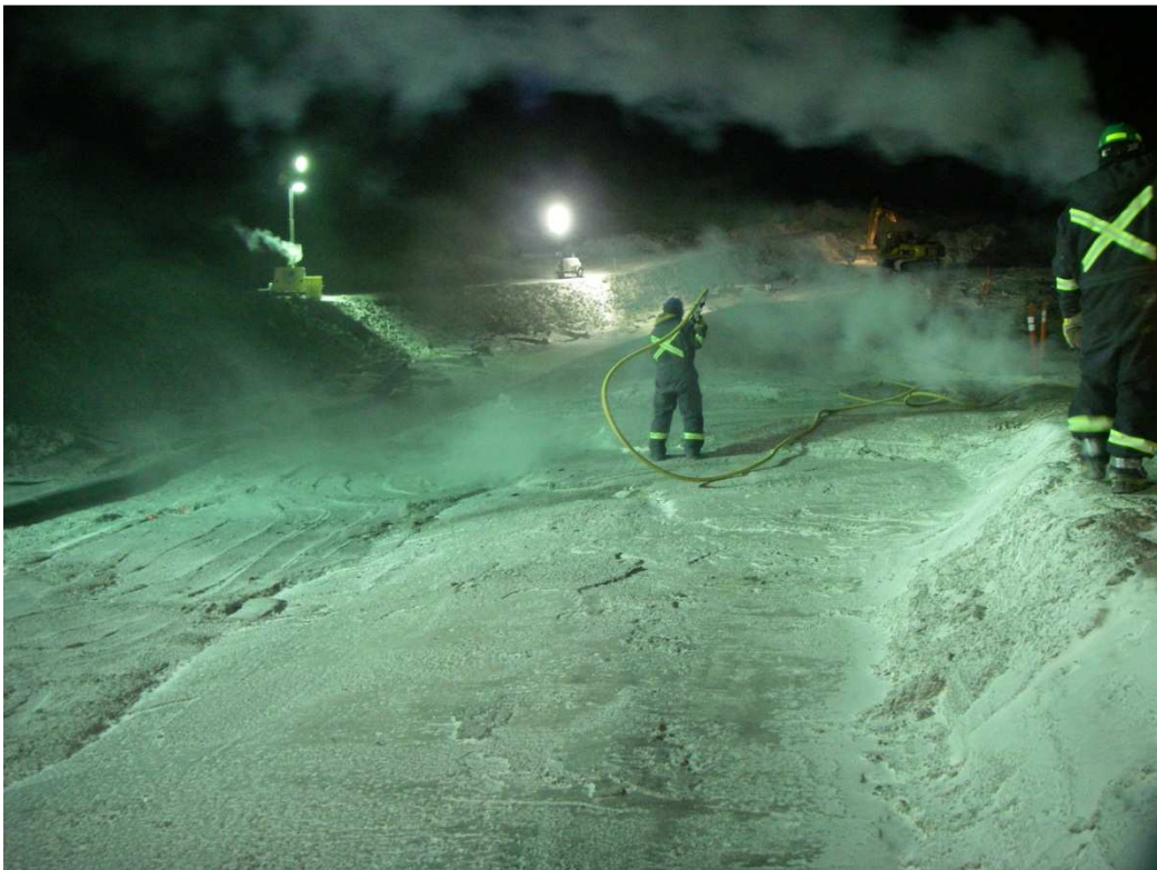
Photo 9: Worker cleaning the frozen core in preparation for placement on night shift.
